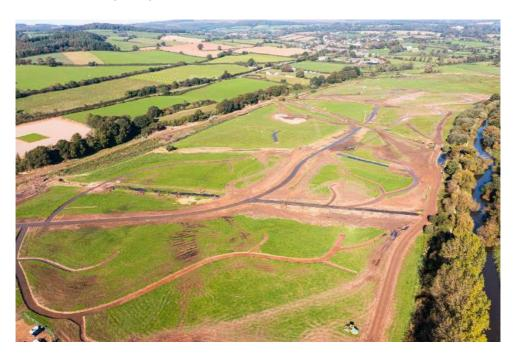
Excavation of the network at the northern end of the site – north of South Farm Road – is now largely completed. Next spring, creeks will be excavated in the south of the site, connecting to the north under the new South Farm Road bridge.
