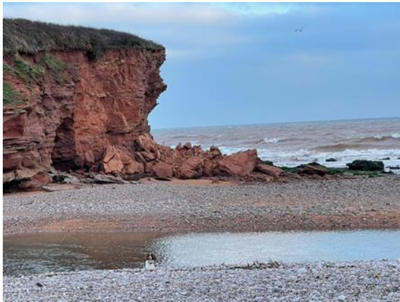
Cliff erosion at Otter Head. Ed
